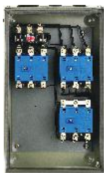
Interior View of ML SASD
