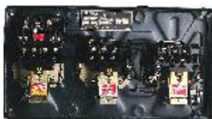
Interior View of MK1 FASD
