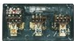
Interior View of MK2 FASD
