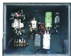
Interior View of MR-G2W
